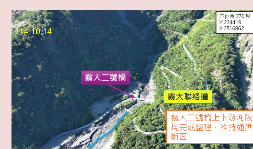
Wuda No. 2 Bridge
